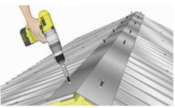
**66.** Place 3 **Metal Ridge Caps** onto apex of roof. Evenly space from front to back of your shed, Metal Ridge Caps will oveerlap eachother. Overhang the cap approximately 1" - 2" past each end. When **Metal Ridge Caps** are correctly positioned, secure with **12 - 2" Metal Ridge Screws** (6 per side). Screw into center of final **Batten**. Do not overtighten!
