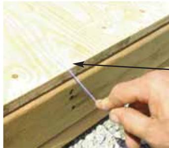
**Hint:** Use a chalk line to mark location of floor joists to determine screw placement.
