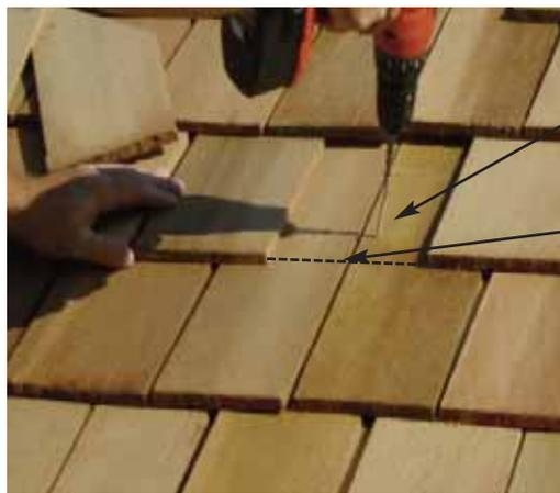
**52.** Screw first filler shingle down to rafters using 1 - 2 1/2" screw per panel (2 in total). Make sure to screw into both rafters.
