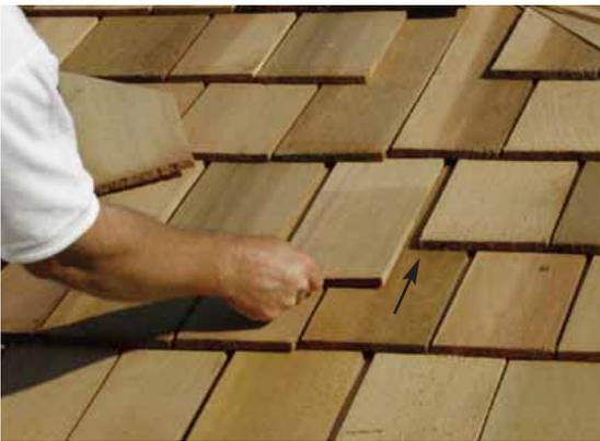
**53.** Slide in another Long Filler Shingle and attach as per **Step 52**. On your last row of shingles, the filler shingle is precut to fit properly. Attach to roof with 2 Shingle Nails per shingle.
