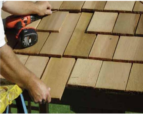
**51.** Roof **Filler Shingles** are included to cover roof seams. Starting at the bottom, slide the first Long shingle in until flush with other bottom shingles.
