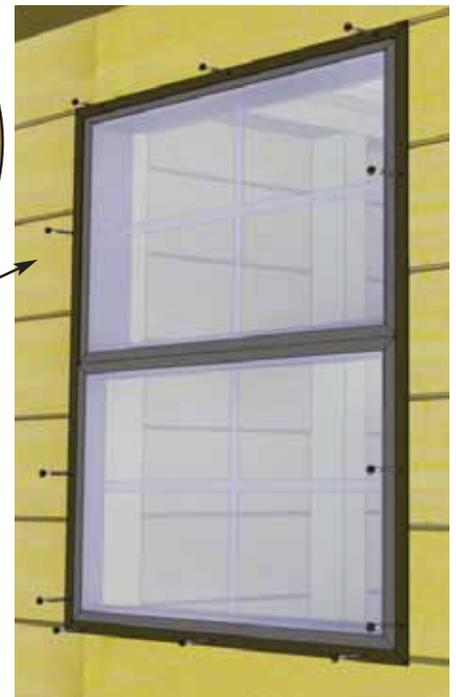
**59.** To reduce possible water from penetrating into the window cavity, caulk gap on both sides of window opening prior to installing **Window Insert**. Position insert in cavity and screw with 6 - 1 1/4" **Screws**.
