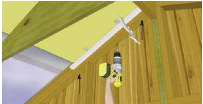
**1.** Locate long and short cleats. Position cleat on top of gable framing tight against rafter. Clamp and screw to gable frame with **3 - 2 1/2" screws** in short cleat and **3 - 2 1/2" screws** in long cleat.
