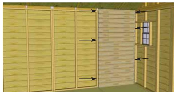
**16.** Locate Right Solid Wall Panel (42 3/4" wide). The right panel will have wall siding recessed on the right side as illustrated above. Position on wall studs and secure with **6 - 1 1/4" screws**.
