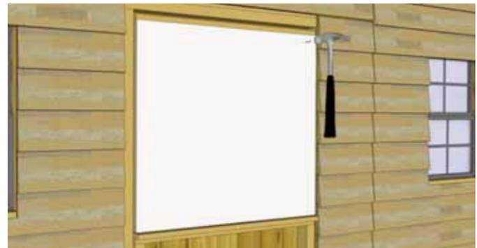
**29.** Position top door plywood over door framing. Confirm it is evenly spaced on door framing and attach with **12 - 1 1/2" finishing nails**.
