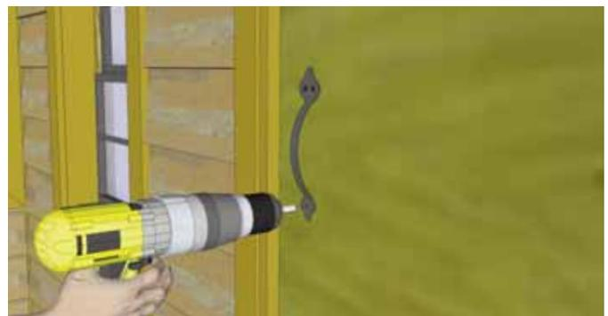
**43.** Attach barrel bolt to door plywood. Male bolt attached to top while female to bottom door. Attach door handle to top door. Use 3/4" black headed screws for both pieces.
