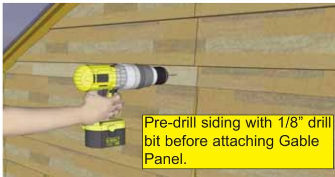
Pre-drill siding with 1/8" drill bit before attaching Gable Panel.
