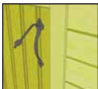
B. Insert Thumb Piece through door hole.
