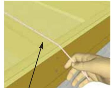
**Hint:** Use a chalk line to mark location of floor joists to determine screw placement.
