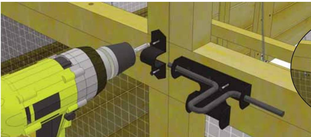
**10.** Attach Black Barrel Bolt to door and panel frame using **6 - 3/4" Black Screws**. Note how female part of Barrel Bolt is positioned higher than male. Do a dry run first to position Barrel Bolt correctly, then attach. Pre-drill with 1/8" drill bit to prevent wood from splitting.
